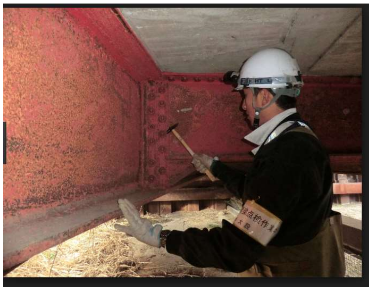
図 1 Hammer test of bridge
